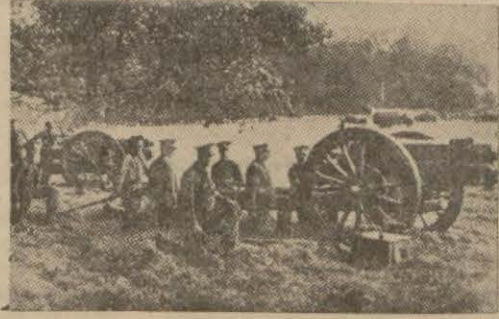
Tank ve batarya
